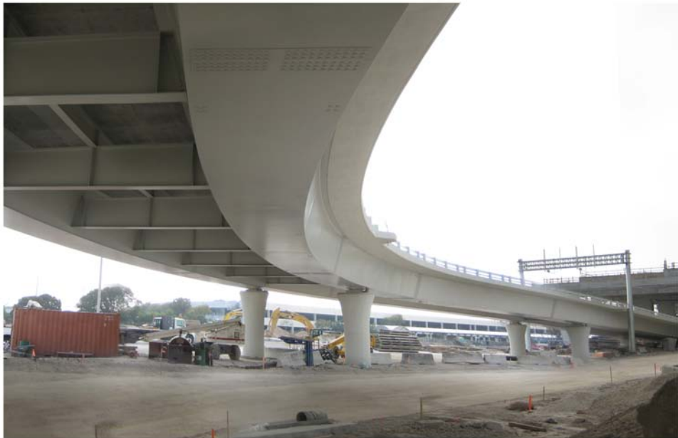
Miami Intermodal Center Construction: Progress Photo February 13, 2009 Rental Car Center (RCC): FM # 249937-5 / MTAR FM: # 249937-4 View of MIC Terminal Access Road Bridge 10-A
