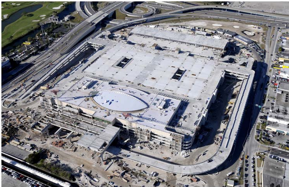
Miami Intermodal Center Construction: Progress Photo January 27, 2009 Rental Car Center (RCC): FM # 249937-5 Southwest View of RCC Construction Site
