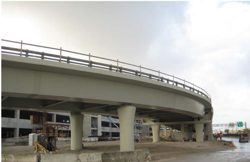
Miami Intermodal Center Construction: Progress Photo January 27, 2009 Rental Car Center (RCC): FM # 249937-5 / MTAR FM: # 249937-4 View of MIC Terminal Access Road Bridge 10-A
