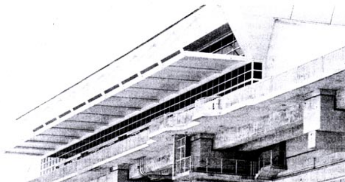
One of four stations for the Sky Train, which is to begin running in September, a respite from long hikes.
