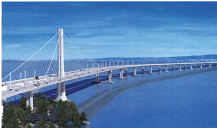
This computer rendering shows the span design of the new San Francisco-Oakland Bay Bridge signature self-anchored suspension bridge, which is approaching $3 billion according to the current cost estimate.
