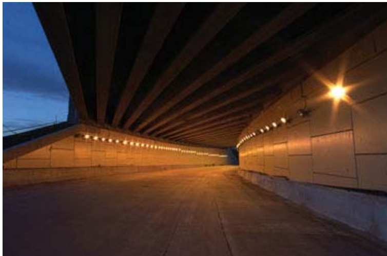
A component of the multimodal T-REX project in Colorado, this new tunnel (shown here at night) carries southbound traffic under the interchange from Interstate 225 to Interstate 25.
