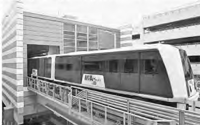
MIA Mover pulls into the terminal at Miami International Airport. It's key to the Miami Intermodal Center.
